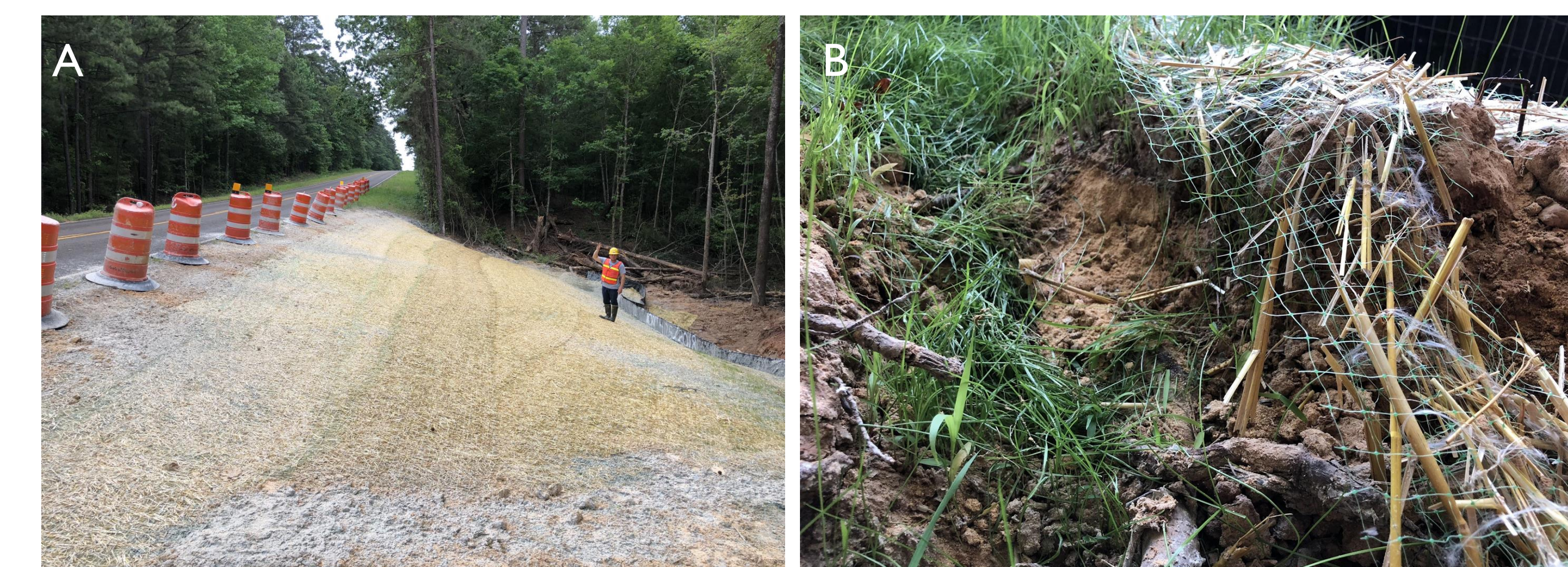
Fig. 7: A) An TXDOT construction site with an ECB installed across the landscape. B) The exposed edge of an ECB S32 DB (2 layer ECB with fused, polypropylene netting).
